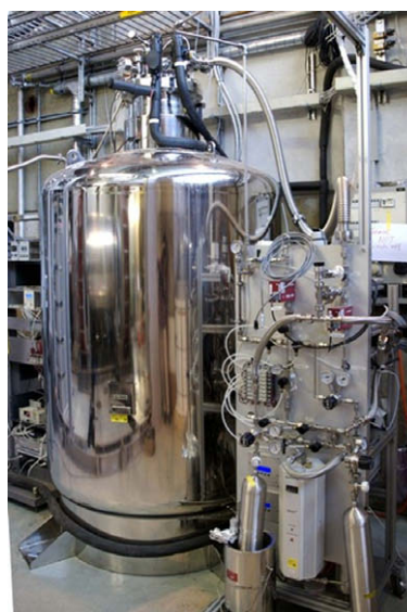
Fig. 3. LXe cryogenic tank with gas purification system.
